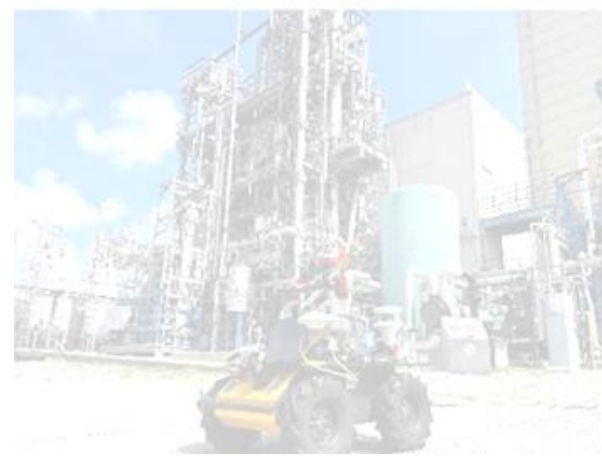
Corrosion Survey, Mitigation & Repair (Industry)
